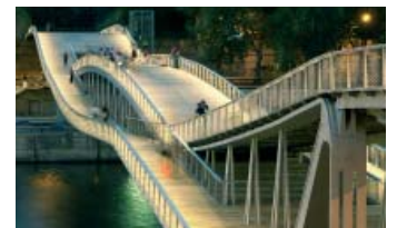
Passerelle Simone-de-Beauvoir, Paris 2006
